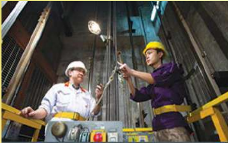
Electrical & Mechanical Engineering and Construction
