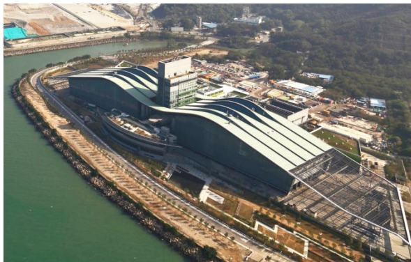
Sludge / Waste Treatment Facilities
