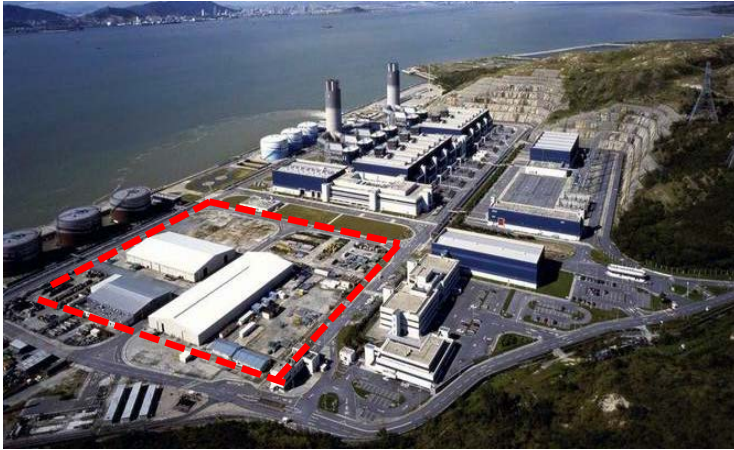
New Combined-Cycle Gas Turbine
