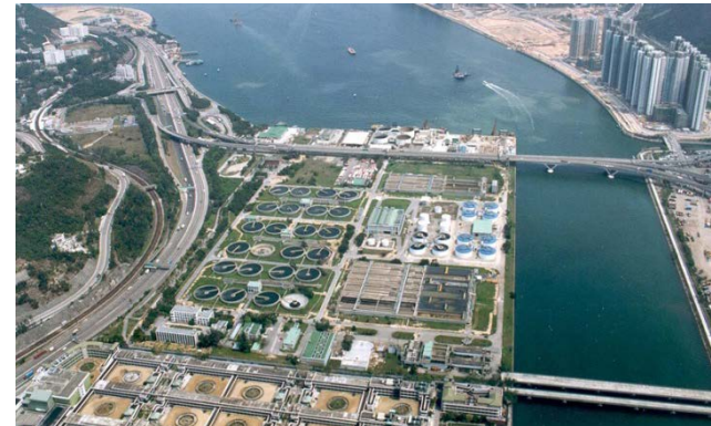
Water / Wastewater Treatment Facilities
